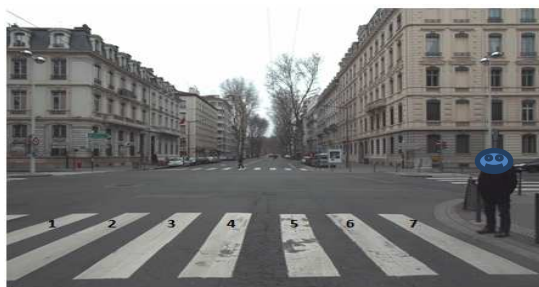
Figure 14 - Example of identified road markings, Lat = 45.7724° and Lon = 4.8431°.
