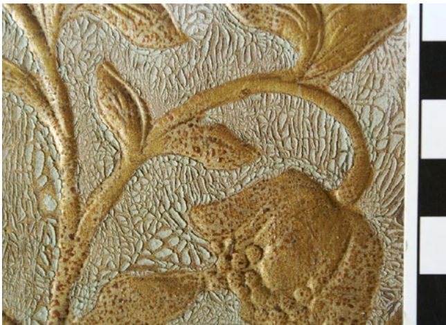
Figure 3: The surface of the blue grey background is cracked and flaking, and in danger of falling off, © Schloss Moritzburg, photo: Gabriele Hilsky
