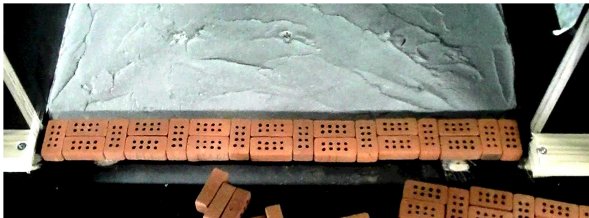
Figure 5. Picture of the assemblage used for each layer: the wall was constructed layer by layer.
