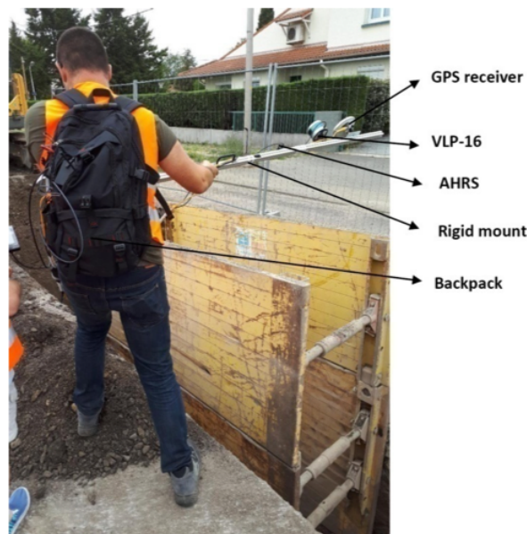
Figure 2. Scanning a ditch using the portable 3D data acquisition system.
