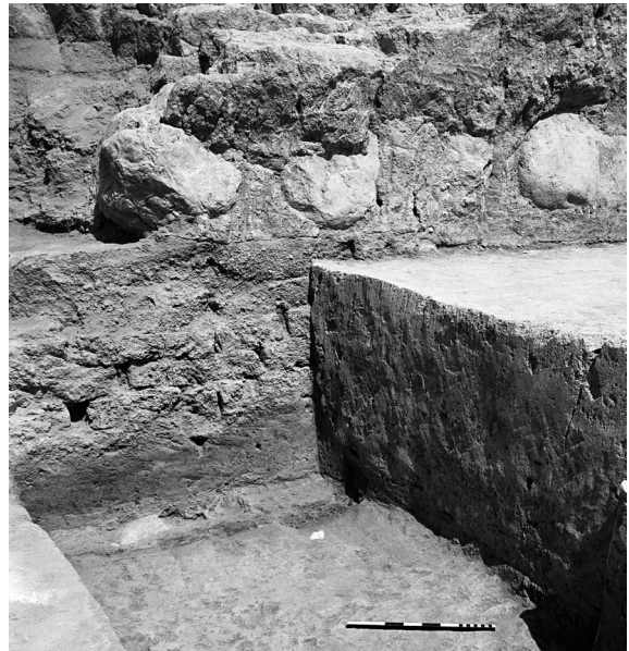
Fig. 4 – Foundations of the outer coffer-work wall of the high terrace, in the southwestern area, view from the SSW, 1971 (photo: Mission archéologique française de Tureng Tépe).
