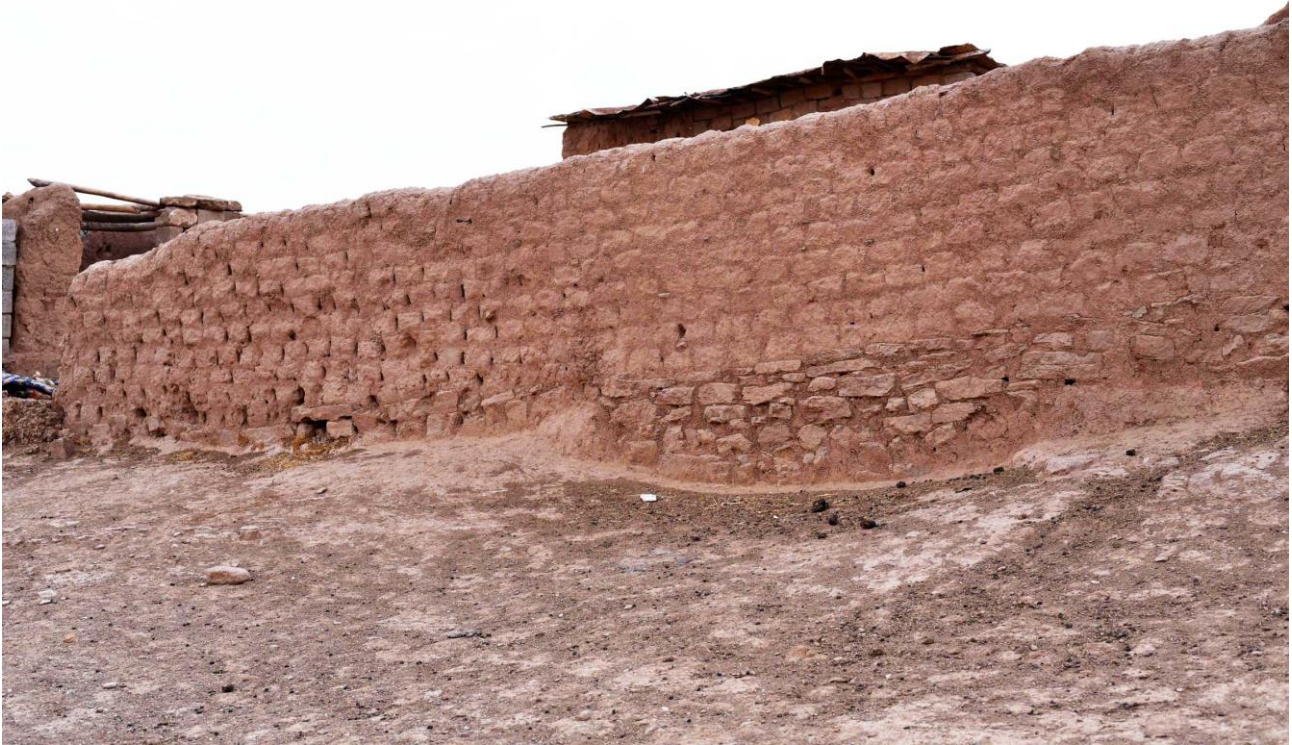
Fig. 13 – Mud brick wall with stone foundations in Kurata hamlet.
