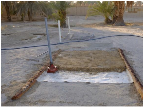
Rammer in metal for pathway compaction (Hili, United Arab Emirates)
