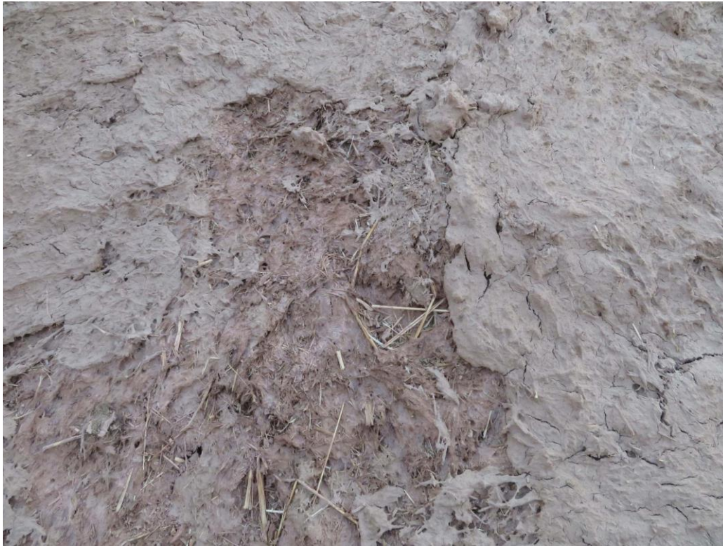
Fig. 10 – Detail of the external layer composed by mud and chopped straw, covering the mound.
