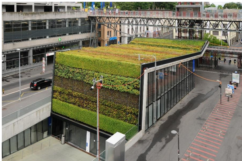
Figure 4: Vegetated roof and walls of the Flon metro station in Lausanne, Switzerland. Architects: Bernard Tschumi Architects and Merlini & Ventura, vegetation: Canevaflor (photo Jean-Luc Bertrand-Krajewski).
