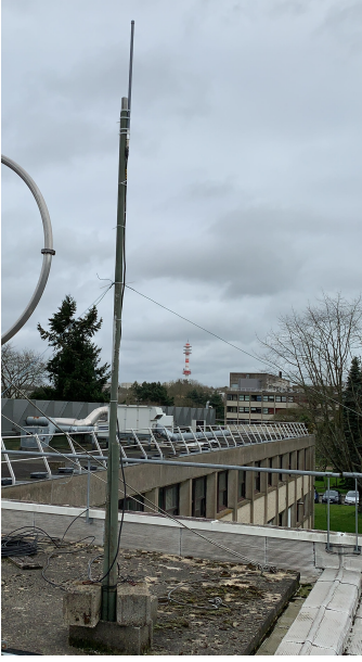
(a) Position of the Rx monopole antenna fixed on the roof.
