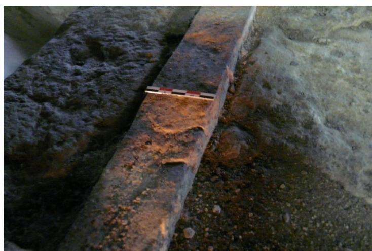
Figure 3. Welding line observed on TN3 tie-rod.
