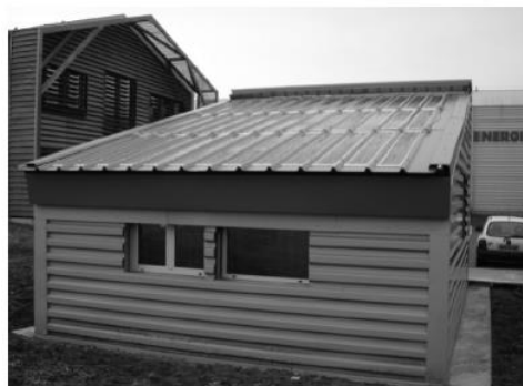
Figure 1. The roof-integrated PVT/air system studied by Assoa and Ménézo [34]. An experimental building at TENESOL company site. Source: Assoa and Ménézo [34].
