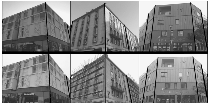
Figure 9. Building contour detection in good and bad weather.
