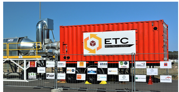
Fig. 1. EcoStock ® of 4 MWh th ( D = 2m and L = 4m ).
