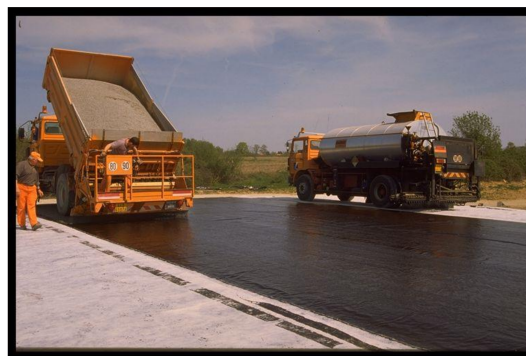
Figure 5. Placement of the 3-layer asphalt wearing.
