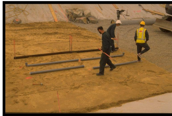
Figure 10. Placement of one of the pipe series in the limestone section.
