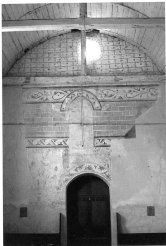
FIG. 10 Ponchon (Oise), parish church, west nave wall. (Photograph: Géraldine Victoir)
