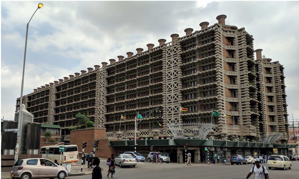
Figure 2. Eastgate Centre, Harare (Image source : Pierre Côté, EAUL, 2018)
