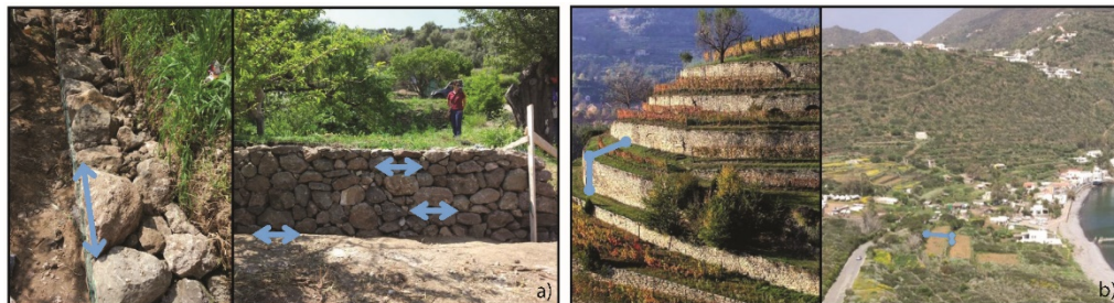
Figure 1. Dry-stone walls (a) and terraces (b). Select building features are highlighted in blue. According to traditional construction techniques, larger stone sides face the outer part of walls (a). Different heights and widths of agricultural terraces determine the root zone and the volume available for water storage (Photo: Stefano Basso).
