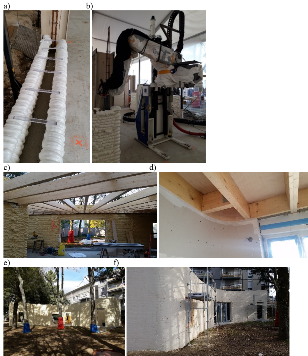
Fig. 7. The construction site of Yhnova™ – a) Deposition of the 6 first layers on the slab showing the reinforcement bars – b) Deposition of PU showing the AGV, the PAA and the protective tent – c) Timber frame for the roof – d) Inner curved plaster boards – e) Outer view of the walls – f) View of the wall covered with external coating.
