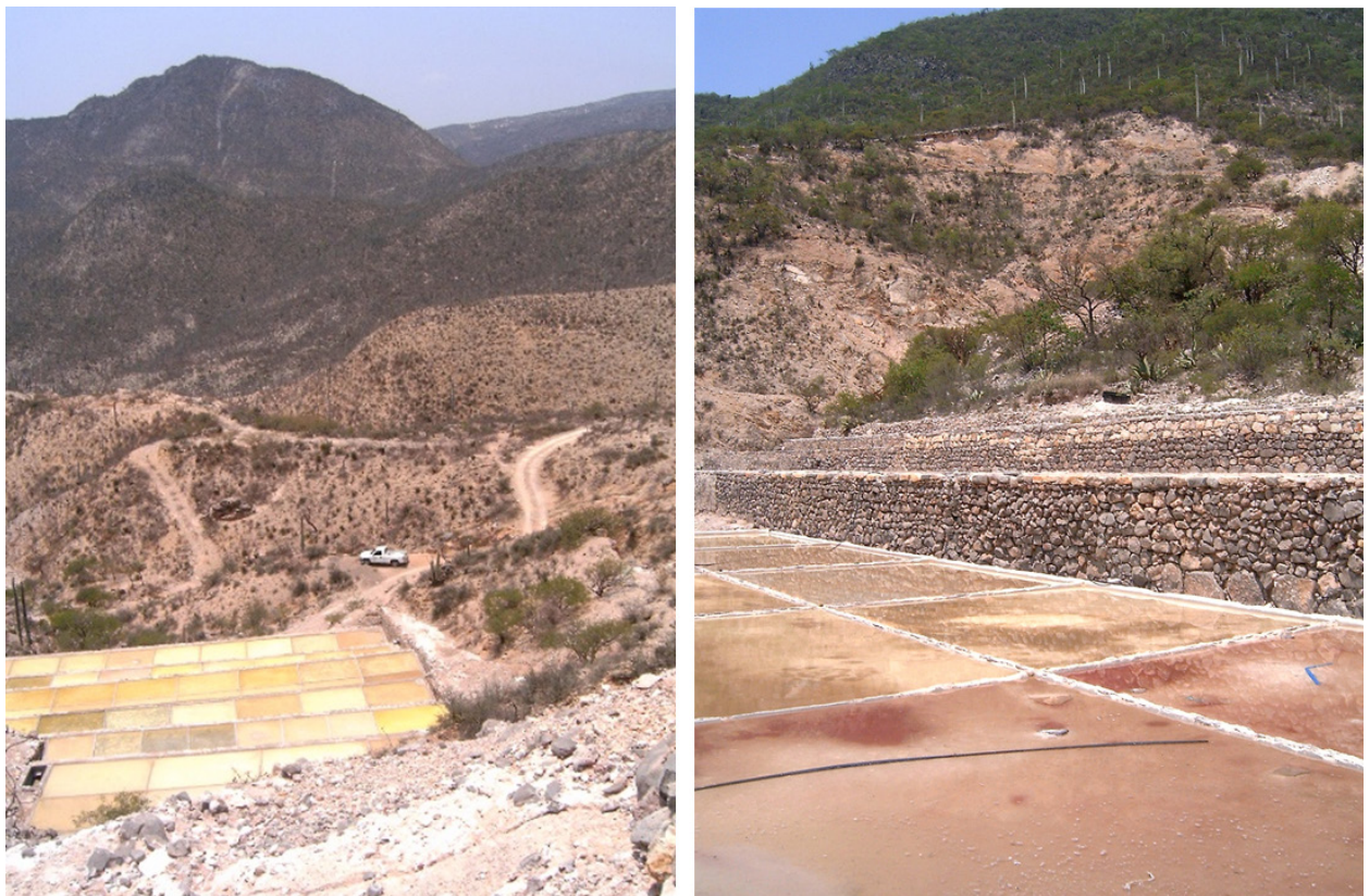
Figure 5. Example of saltworks located in ravines and steep slopes, and the use of limestones to build terraces for evaporation ponds, Salinas Miahuatepec, Zapotitlán, Puebla (Photos by B. Castellón).
