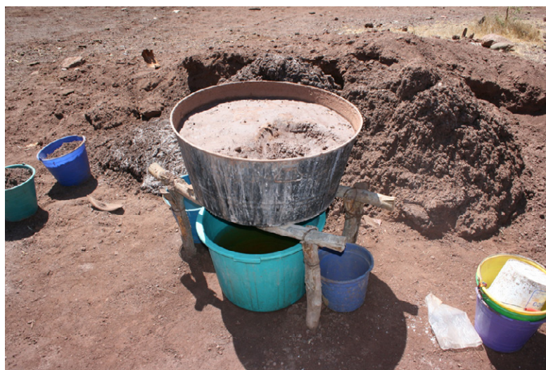
Figure 8. El Salitre, Guerrero. Small filtering mechanism for leaching of salty soils in March 2009 (Photo by B. Castellón).
