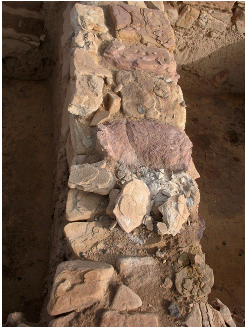
Fig. 11. Top of a sandstone wall foundation. The stones are loosened and broken.
