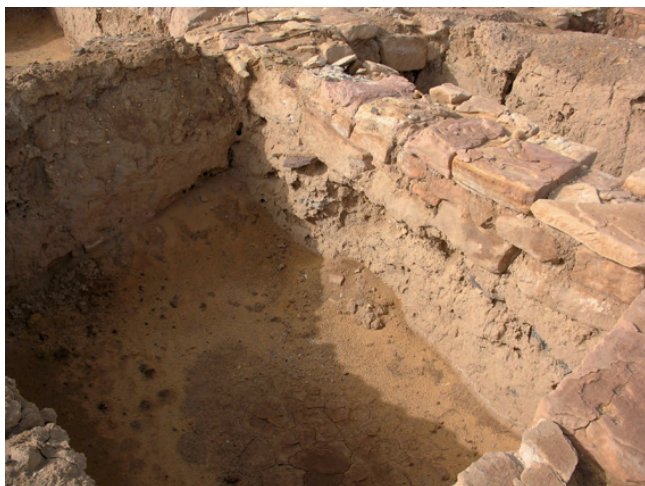
Fig. 32. Room 5, east wall, undermined wall.
