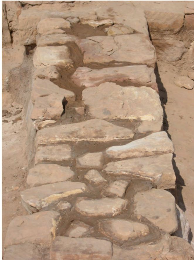
Fig. 27. The joints of the top of the wall have been filled with mortar. Some of the missing parts have been rebuilt with the same materials as those used in antiquity.
