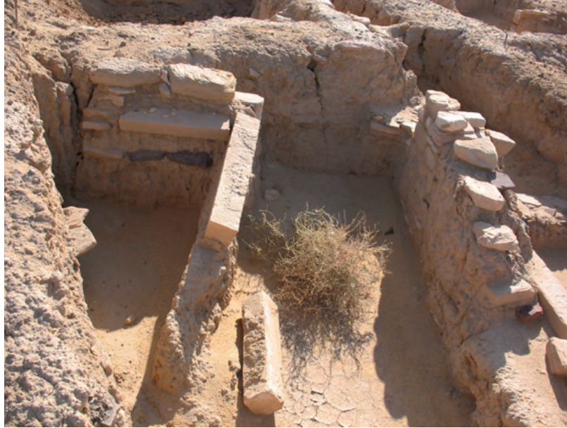
Fig. 10. Undermining below the foundation of the walls leads to their weakening and even to their collapse.
