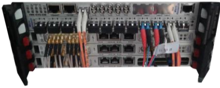
Figure 4: Example of VME rack used.
