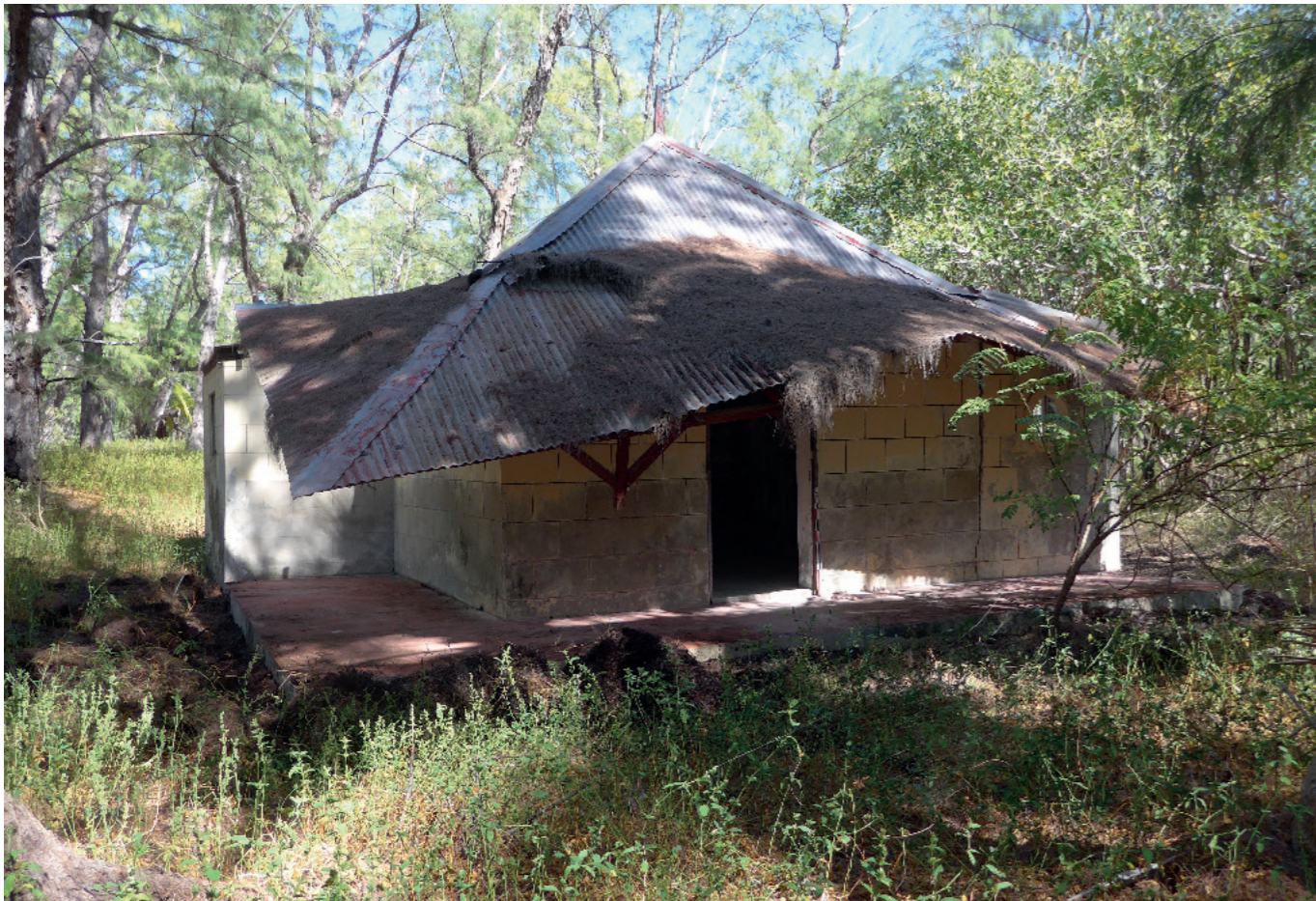
[Fig. 6] : Batiment 2 (photo V. Motte)
