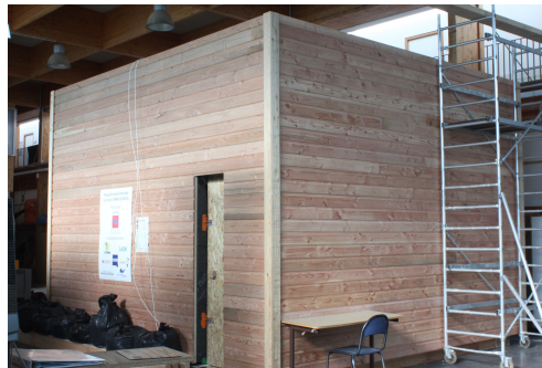
FIGURE 2 – Full scale experimental mock up of VIBRACOUBOIS project.
