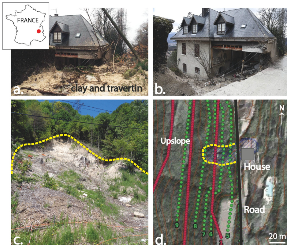
Fig. 1. The shallow landslide of Claix (Isère, France) of December 30, 2017. a. Clayey and travertine-type materials have crossed the road and partly destroyed a house killing a person during the night (ph. G. Guais; December 30, 2017). b. State of the building after clearing of the mud (ph.: S. Gominet – IRMa; January 03, 2018). c. Detachment scar of the landslide on the June 19, 2018. Yellow dotted line: scar border. In the foreground: cables and electrodes. d. Geophysical profiles and location of the landslide. The dots correspond to the electrodes.
