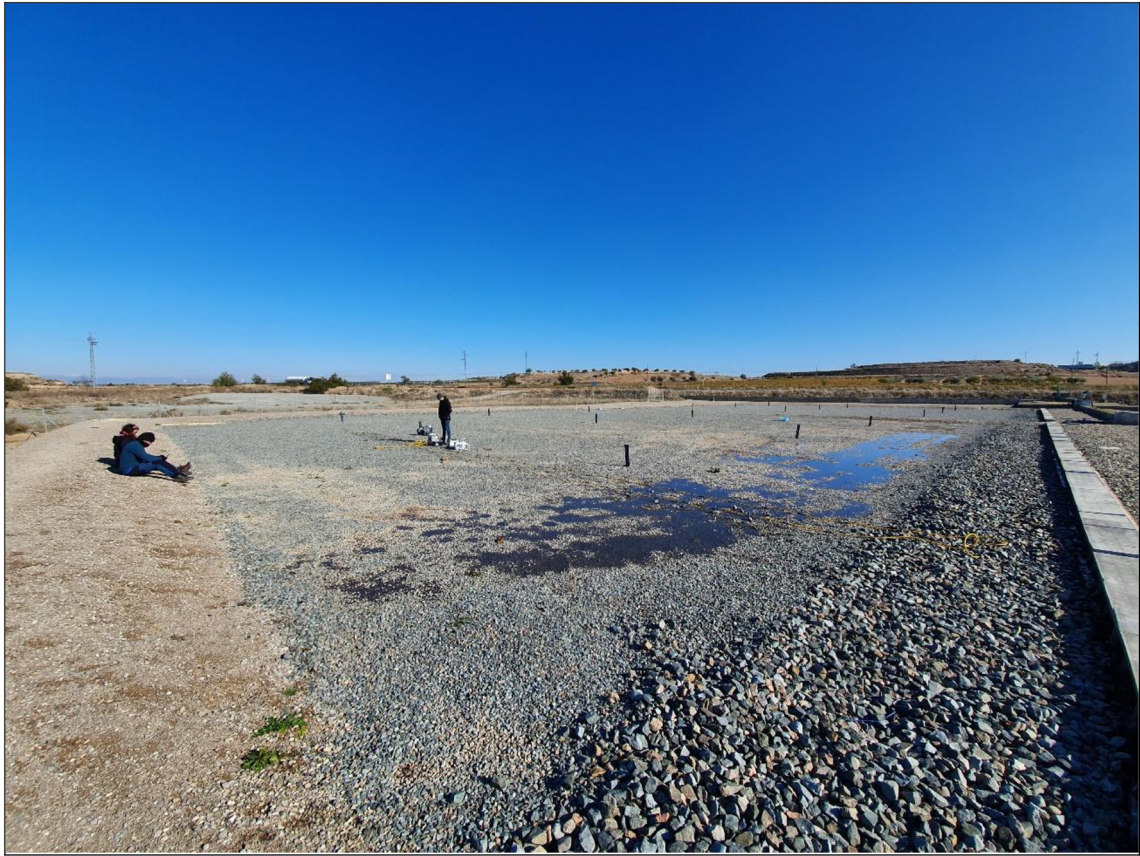
Fig. 7. Picture of the constructed wetland investigated in the present paper. The surface flow can be seen along the water inlet as well as the nine piezometers.
