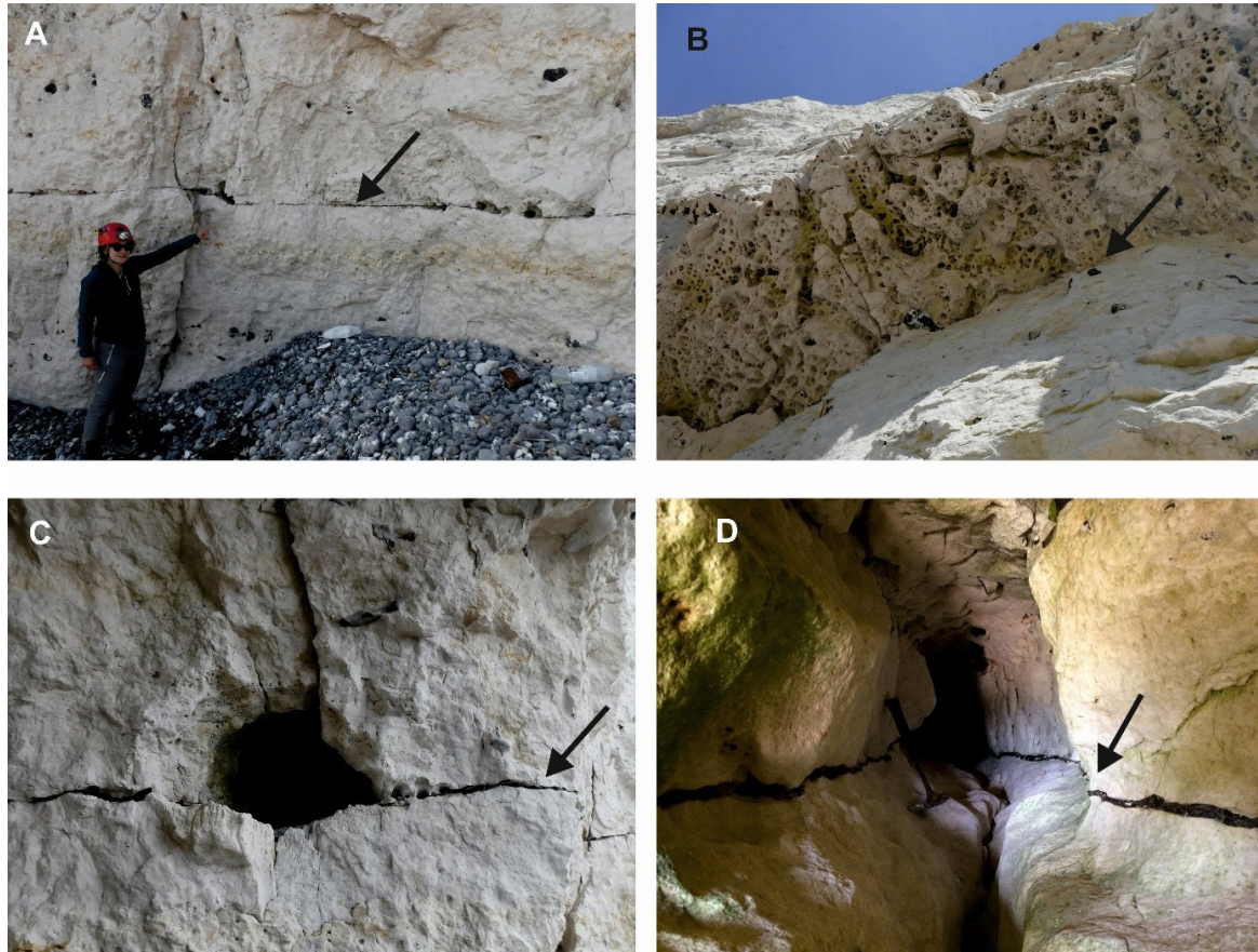
Fig. 12. Dissolutional conduits formed by mixing dissolution above a sheet flint (arrowed). A) St Margaret's Bay, Kent; B) Detail looking up at the underside of a bedding surface (the sheet flint has fallen away) showing a conduit network embedded in a mesh of small dissolutional voids ('tubule karst' of Lamont-Black & Mortimore, 2000), Beachy Head, Sussex; C) St Margaret's Bay, Kent; D) Hope Gap, Seaford Head, Sussex.
