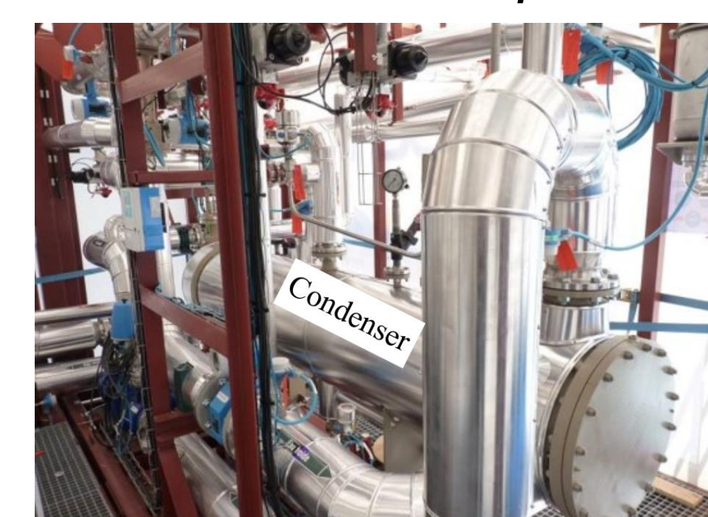
Smooth shell-and-tube Condenser
