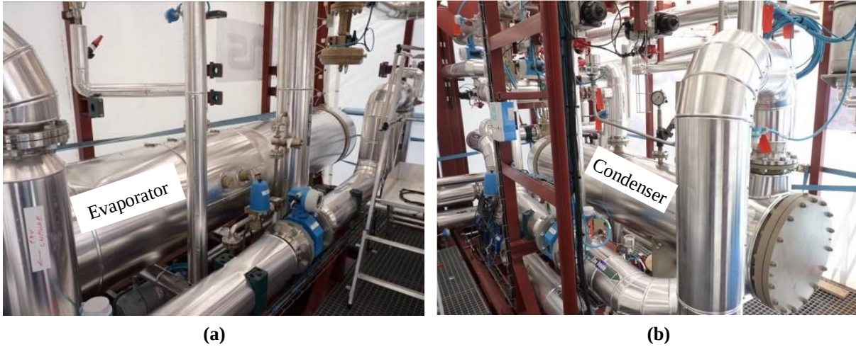
Fig. 5. The flooded shell-and-tube evaporator (a), the shell-and-tube condenser (b)
