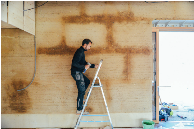
△ Figure 8. Filling joints between prefabricated rammed-earth wall panels. (Credit: designbuildLAB)
