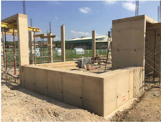
△ Figure 6. North/west corner stem wall and moment frames. (Credit: designbuildLAB)
