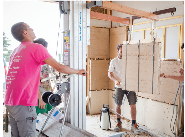
△ Figure 7. Lifting prefabricated rammed-earth wall panels into place. (Credit: Lauriane Lespinasse)
