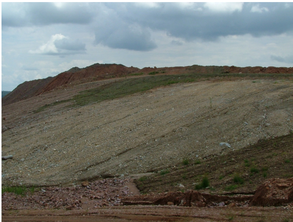
Figure 4. Large-scale earthwork often constitutes the first step in post-mining restoration. In the Katanga copperbelt, Democratic Republic of Congo, various grassland communities occur on outcrops depending on a gradient of copper (Cu) and cobalt (Co) concentrations. The image shows a post-mining restoration site where a hill was re-shaped to create the template for restored grassland communities. The hill comprises relatively high Cu-Co concentration subsoil. A small area of high Cu-Co concentration topsoil was spread on which vegetation has already established (photo credit S Le Stradic, Technische Universität München, Germany).
