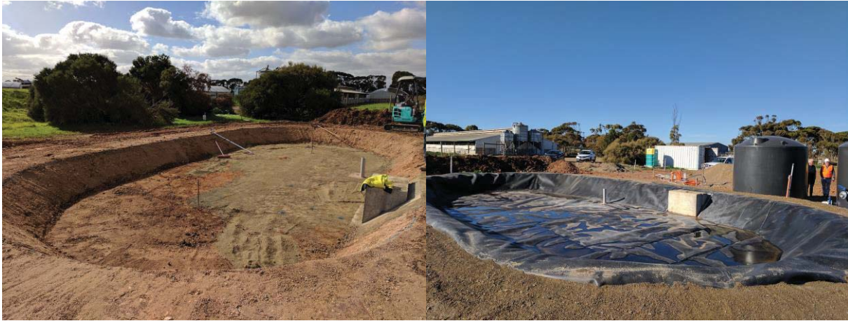
Plate 2 The outline of high rate algal pond with the completed dam wall and pond liner (June 2017).
