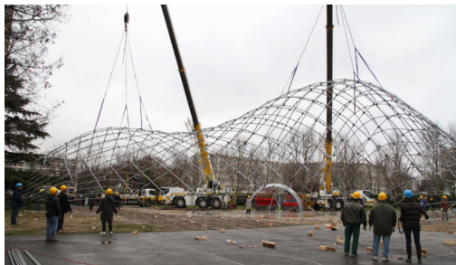
(a) Beam grid of the Ephemeral Cathedral in Créteil, France [1] (Photo credits: thinkshell.fr)
