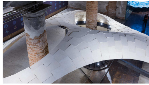
(b) Voussoir tessellation of the Armadillo Vault in Venice, Italy [2] (Photo credits: Iwan Baan)
