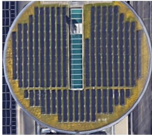
Figure 9: Aerial view of a flat roof implementation of PV systems on a building in Geneva.
