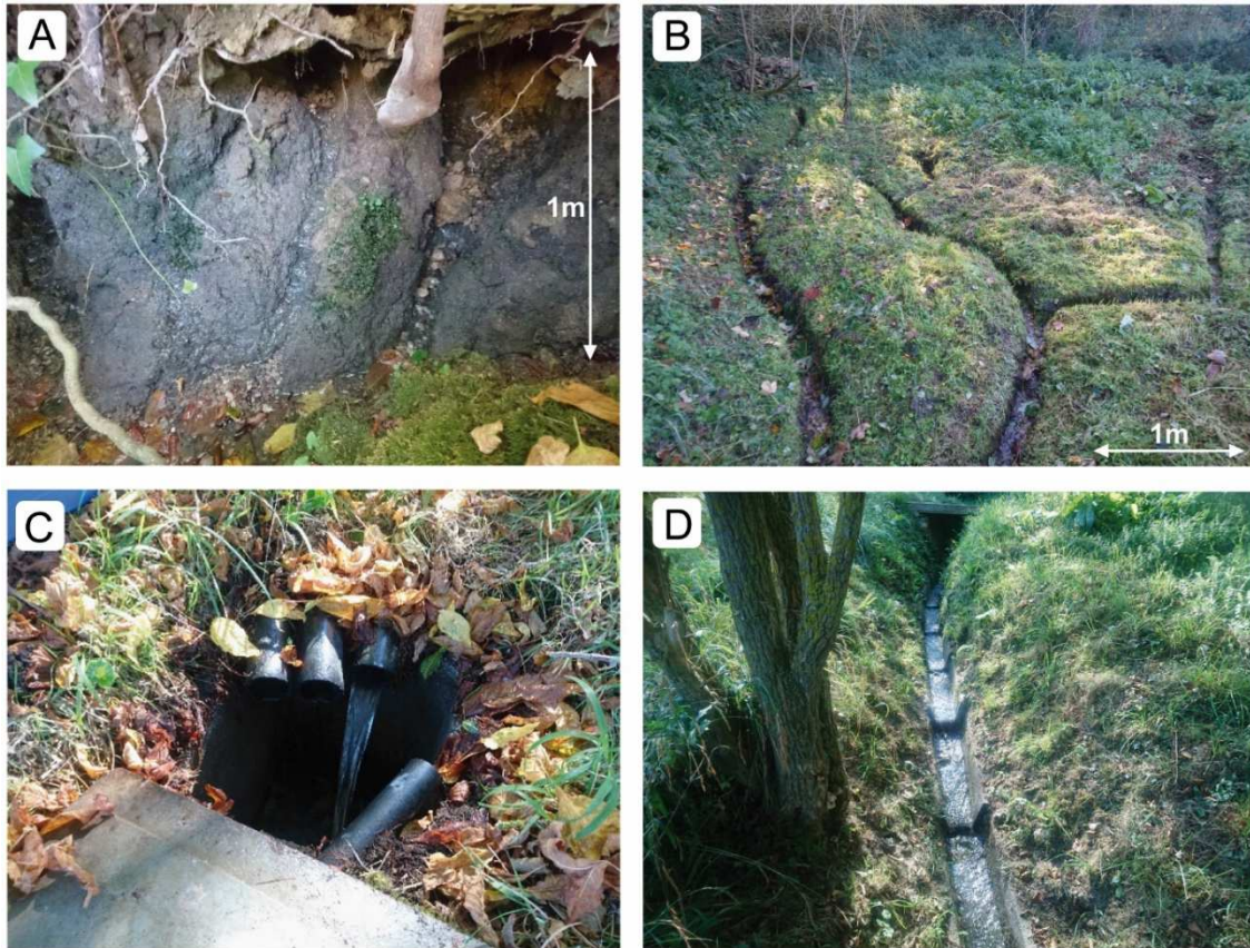
384 Fig. 10 – A: Natural spring from the Cenomanian chalk at the basis of a five-metre-deep scarp; B: Trenches dug in the soil to 385 channel and drain surface waters; C: Water arrivals from four drainage pipes in a concrete manhole for recovery in a larger 386 pipe; D: Open trench built with overlapped precast concrete elements
