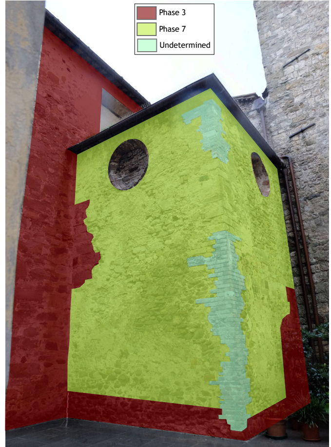
Figure 17: The north lateral chapel. The first phase of the building is colored in red. The green part corresponds to a repair of the first phase.
