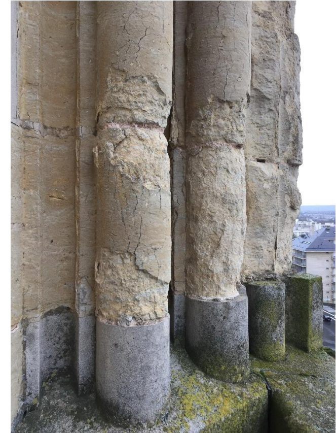
Picture of weathered stones and restored stones on the Basilica.
