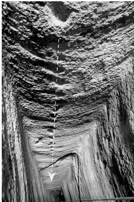
Figure 6. Laurion. Spitharoussi sector. Quadrangular section shafts. Grooves on walls: timber remains of ventilation system seen from the surface. (Spi 6)
