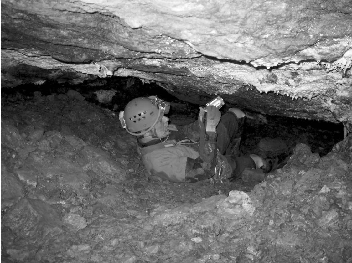
Figure 14. Laurion. Spitharopoussi sector – Spi 18. Deep works in the Third Contact. Ancient mining works around – 80m. Access lane and accumulation of waste (backfilling)
