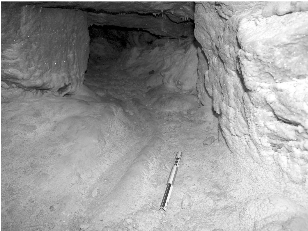
Figure 20. Laurion. Spitharopoussi Plateau. Spi 49 – Deep works in the Third Contact. Clear traces of dragging on the ground fossilized by the calcite. Junction gallery between two work zones
