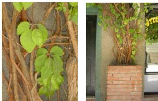
Fig.4. Parthenocissus quinquefolia covering the building "A"
