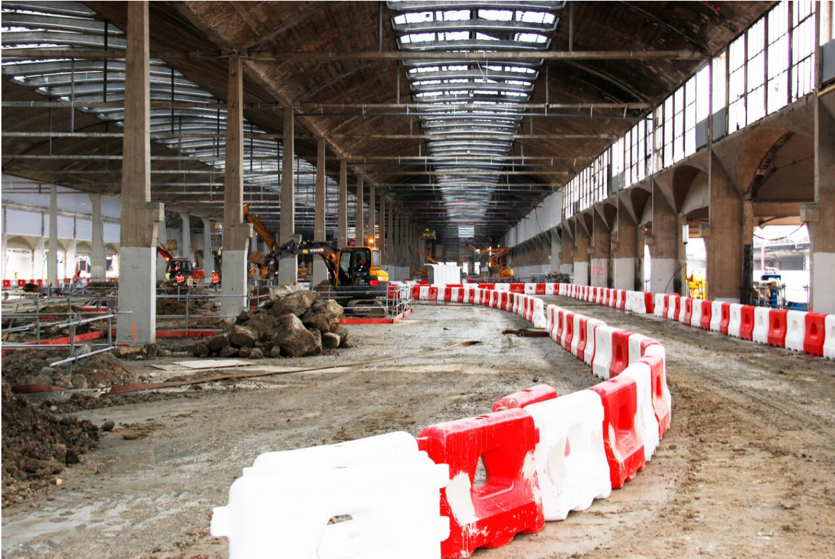
Chantier Hall Fressinet - Paris
