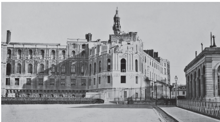
Fig. 9: Restauration du château de Saint-Germain-en-Laye. Charles Marvilles, 1862. ©MAN
