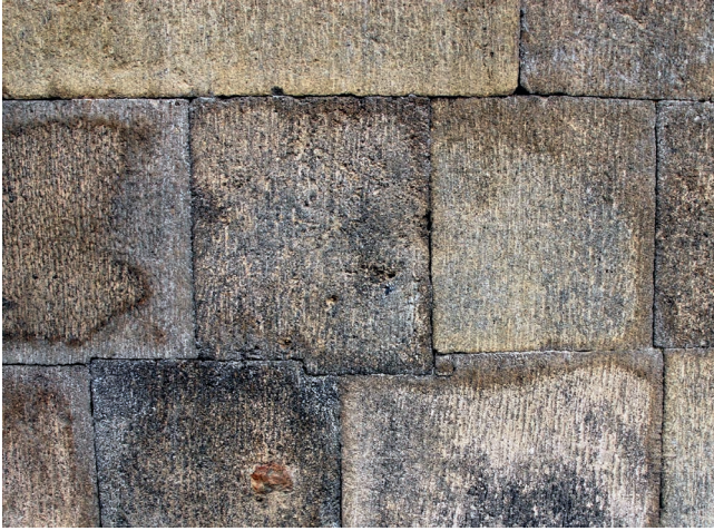
Fig. 4 — Candi Kimpulan. Main temple. Detail of the stereotomy (photo: V. Degroot/EFEO).
