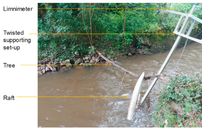
Fig. 12. View from the bank before reparation work.
