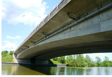
Figure 1. View of PI-57 Bridge.
