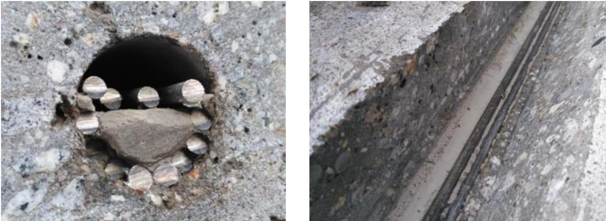
Fig. 5 Front view of prestressing cable (left) and opened cable duct view (right).
