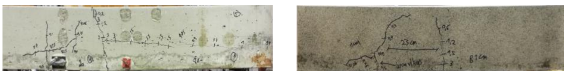
Fig. 5 Picture of cracks developed in the case of 5R1 (left) and 5R2 (right).
