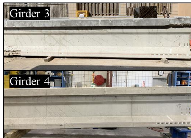
Fig. 4 Crack patterns at ultimate load for Girder 3 and Girder 4
