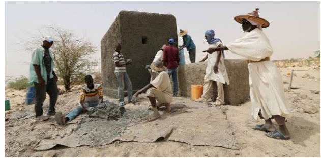
Figure 6. Preparation of mortar for plastering by young masons supervised by the head of the masons' corporation. Mausoleum of Cheik Sidi Ben Amar, April 2015 © Joffroy T. CRAterre.
